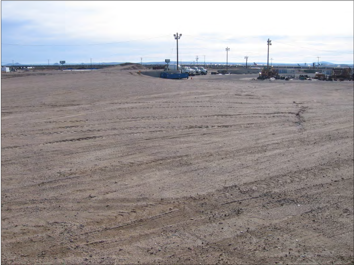
AggreDust installed July 2018. Pictures taken March 2019.
